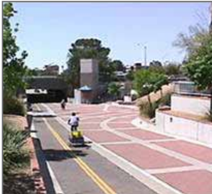
Warren Avenue Underpass
