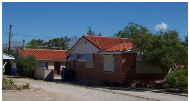
Cross gable roof with clay tile
